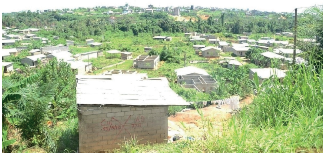
Figure 4. Illegal construction in green areas in Logbessou Quater (Douala). Source: CUD/Tchappi.
