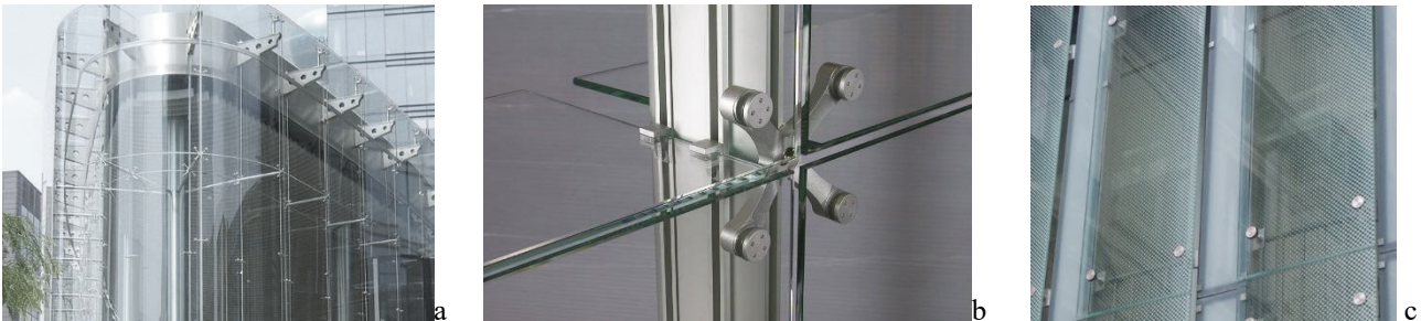
Figs.3 a,b,c : Detail of punctual hanging of glass plates of the most diffuse systems
