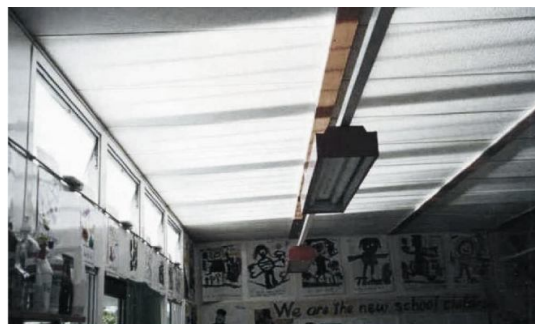
Fig. 17. Application of laser cut panels to South State School environments in Brisbane - Australia
